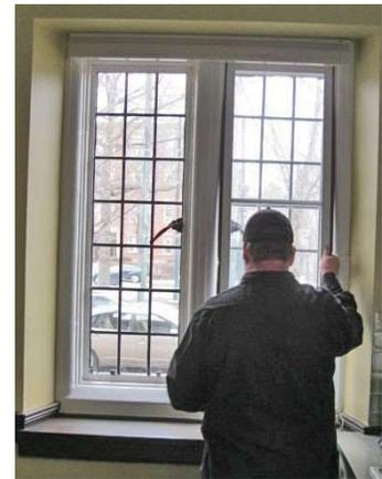
condense on the cold window surface. There are sound-proofing benefits too. The photo at right shows the product being installed on one of those “special/irreplaceable” HOW windows.
