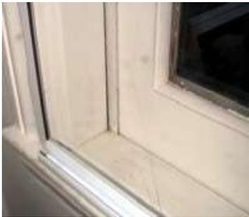
My first window was a hybrid: *magnetic strip* for the sides and top, and a *plastic extrusion* for the bottom, which fits flat on top of a window sill (See photo at left.) Works well, looks good, but somewhat expensive and time-consuming to build.
